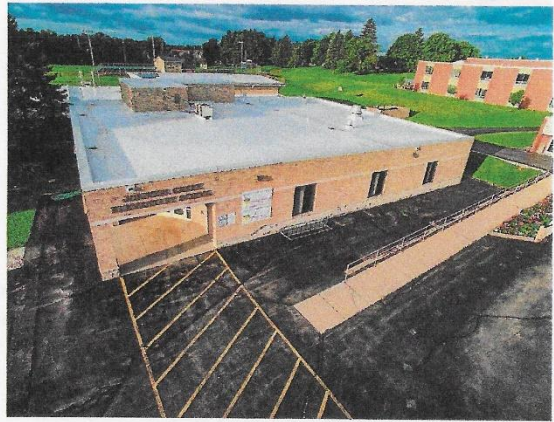
305 Milwaukee St -front entry
