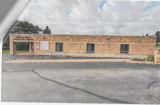
305 Milwaukee St Front entry
